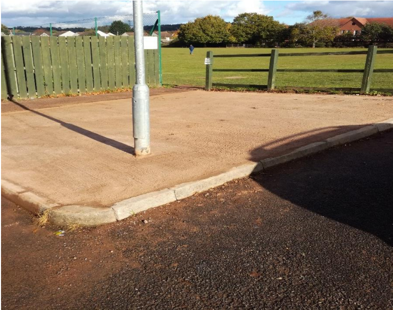
Figure 5 Finished job at Pavilions.
