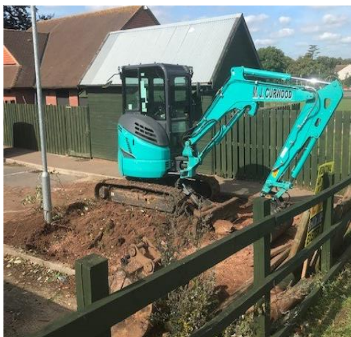
Figure 3 Digging at Pavilions
