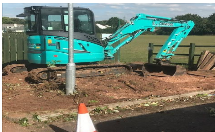
Figure 4 Prep work for concrete
