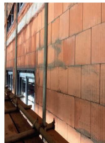
“Porotherm” ceramic wall blocks
