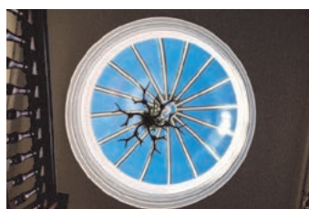
The repaired roof lantern
