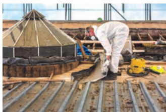
Stripping the Roof
