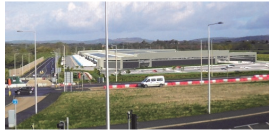
Computer-generated image of the distribution depot viewed from the Clyst Honiton Bypass. It is anticipated construction will commence later this year. (Copyright ©Exeter and East Devon Growth Point 2016)
