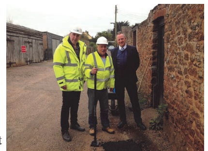
Broadclyst Community Road Warden, Roger Beer (centre) has been 1 of 5 to trial the instant pothole repair material
