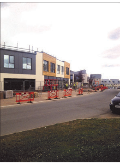
Cranbrook’s Neighbourhood Shops under construction
