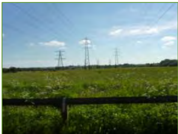
Pylons crossing the Clyst floodplain (CA 2d)
